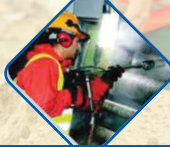
High Pressure Water Jetting Industry
